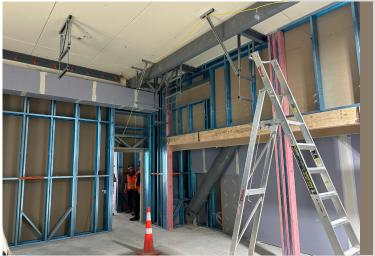
Manufactured in sequence to match the project's construction schedule and delivered flat-packed, each drawing set comes with a unique QR code that links directly to a web-based 3D model viewer. This QR linked to a 3D model viewer that provided everyone onsite with accurate design information on where each component should go and how it was to be installed.
