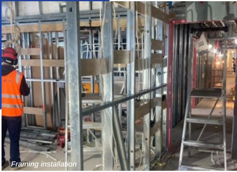
Telescopic framing for Victoria Lane Apartments transported flat-packed to be assembled onsite
